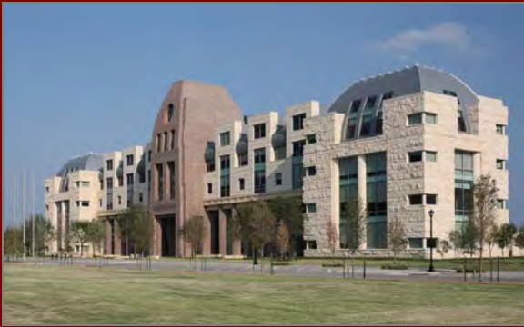
The City of Frisco, Texas recently built a joint City Hall and Library that features green design concepts.
